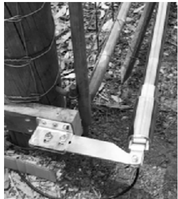
Option A Rear post mounting
